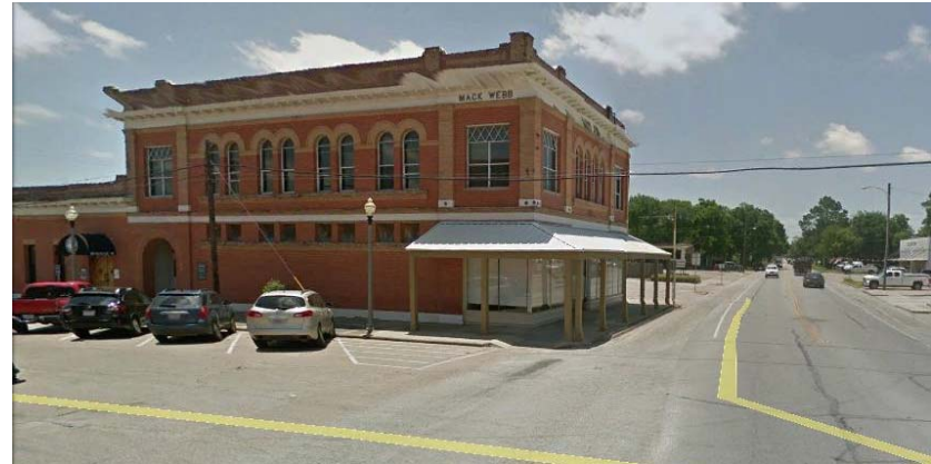
Fig 1.20: A traditional brick cladded building in Downtown El Campo
